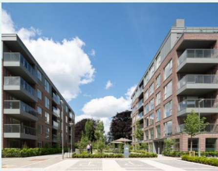
Rostrevor Place, Rathgar 108 apartments Commenced: April 2019 Completed: April 2021
