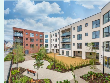
Shackleton Hall, Lucan 60 apartments Commenced: June 2018 Completed: December 2018
