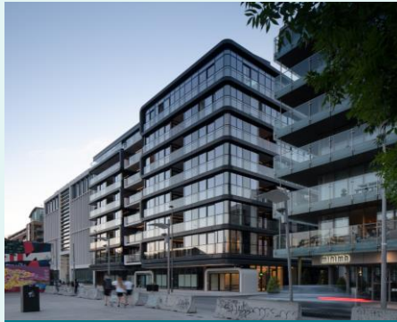
Six Hanover Quay, Dublin 2 120 apartments Commenced: August 2017 Completed: June 2019
